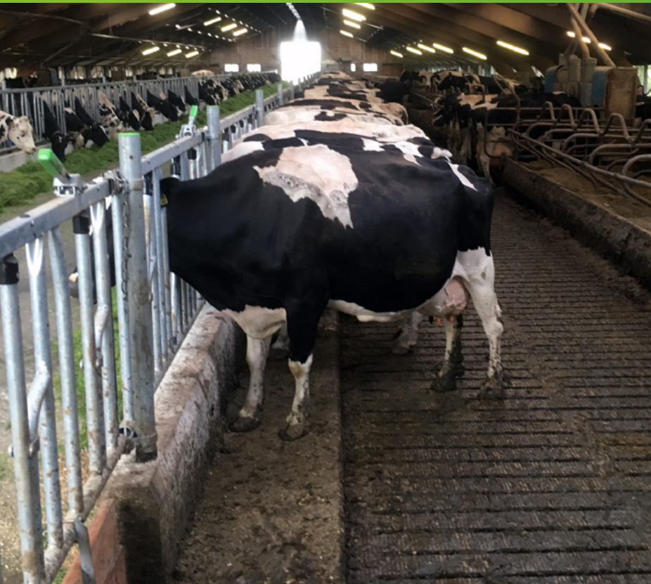
Feed alley after renovation
