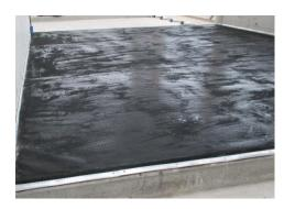
**Step 12:**To finalize the installation, fix the aluminum bars with nails on the extremities of each side.
